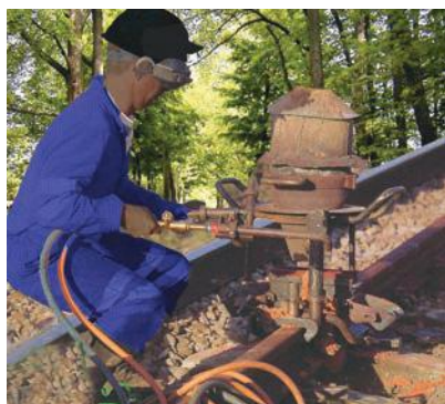
Figure 3.11 Thermit process for joining railway tracks
