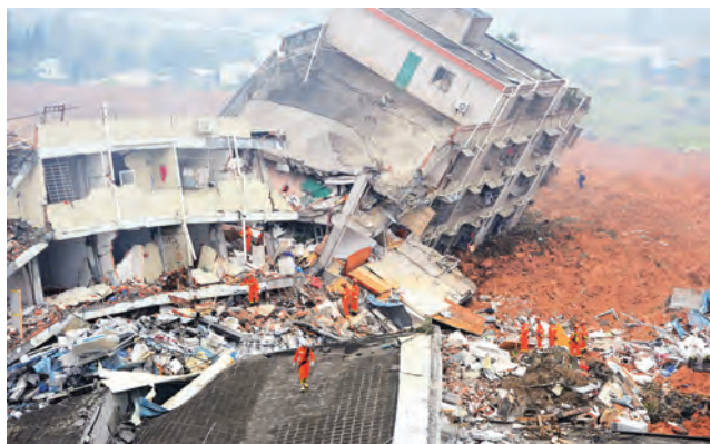
Effect of Earthquake
